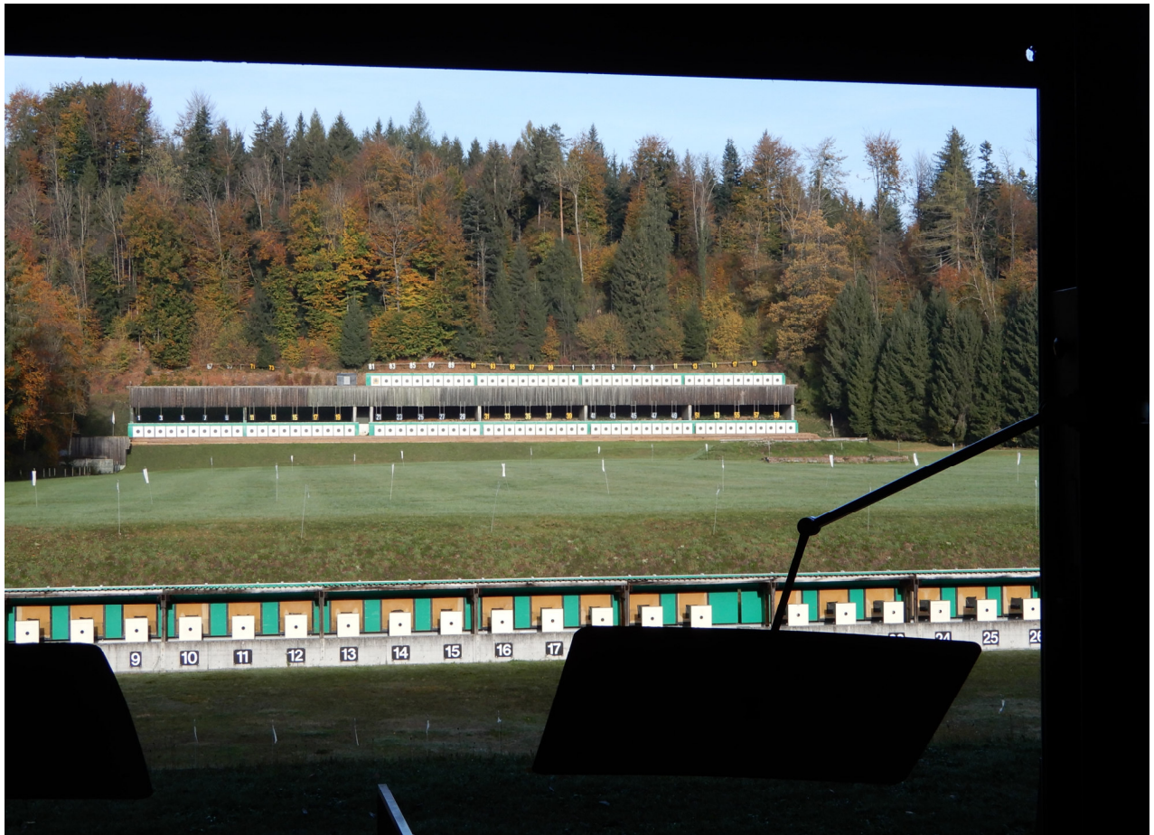
Schiessanlage Guntelsey in Thun
